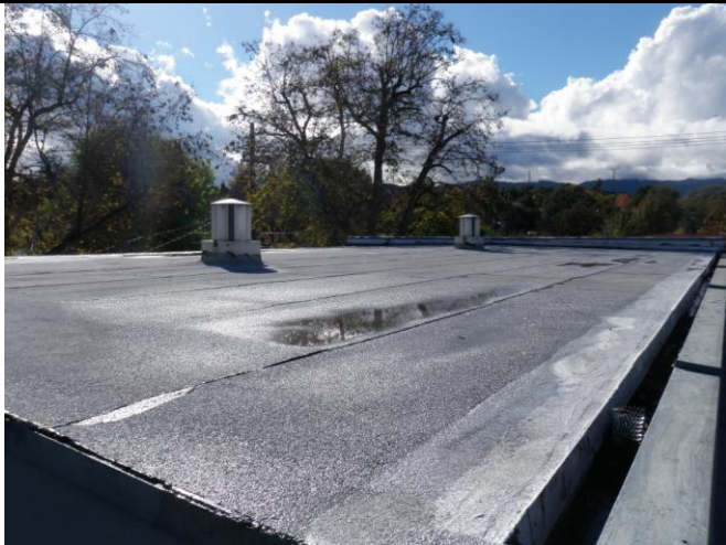
Photo 9: View of the roof
