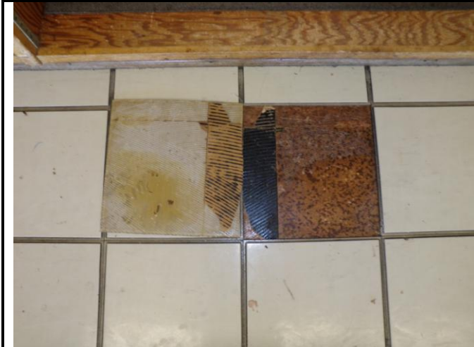
Photo 5: ACM 9x9 vinyl floor tile and mastic under the non-ACM vinyl tile
