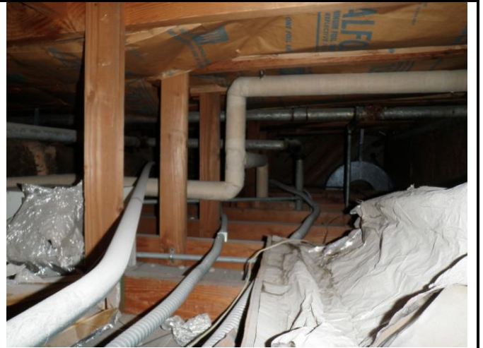
Photo 6: Non-ACM insulation materials in the attic space
