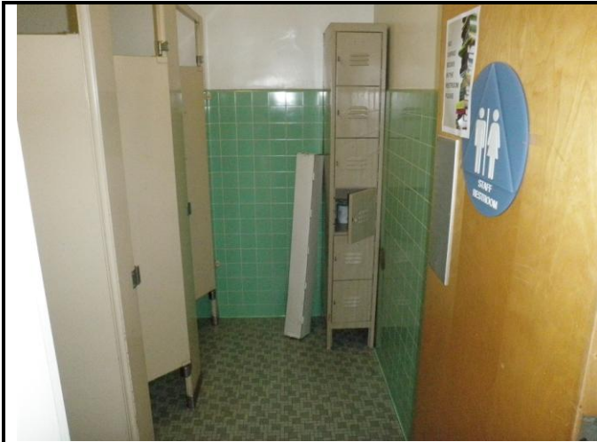
Photo 7: LBP ceramic tile on the walls in the restrooms
