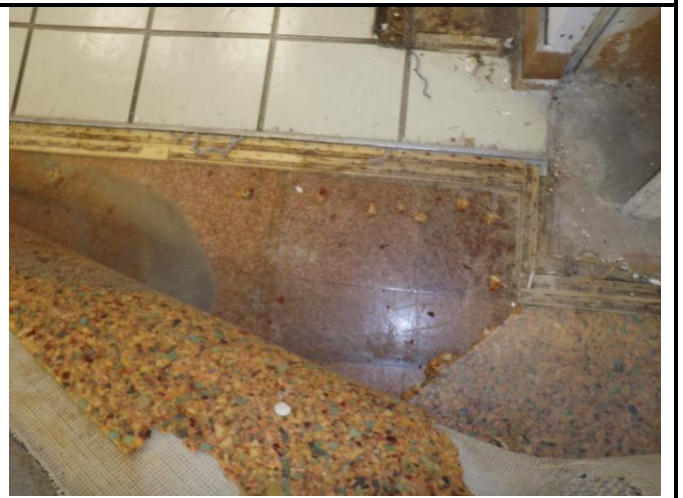
Photo 4: ACM 9x9 vinyl floor tile under the carpet
