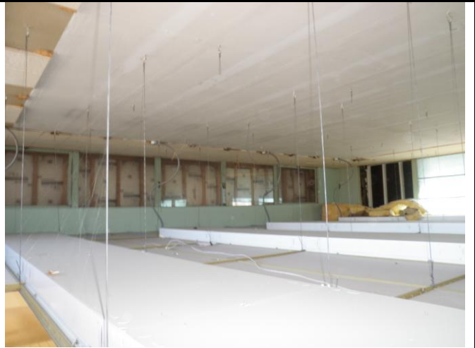
Photo 12: View of the ceiling space above the drop ceiling
